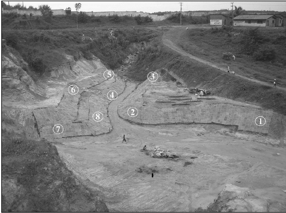
Fig. 4 Rehabilitated areas with cover of Buriti geotextiles, Sacavém, São Luís (areas 1–3 were constructed with men and tractors; upper areas 4–8 were constructed using a tractor) (LAGESOLOS 2008)
