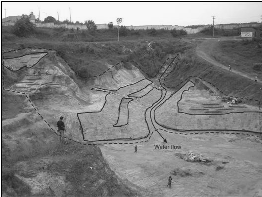
Fig. 5 Continuous lines areas rehabilitated with Buriți palm mats. Hatched lines the rehabilitated area in Sacavém (LAGESOLOS 2008)
