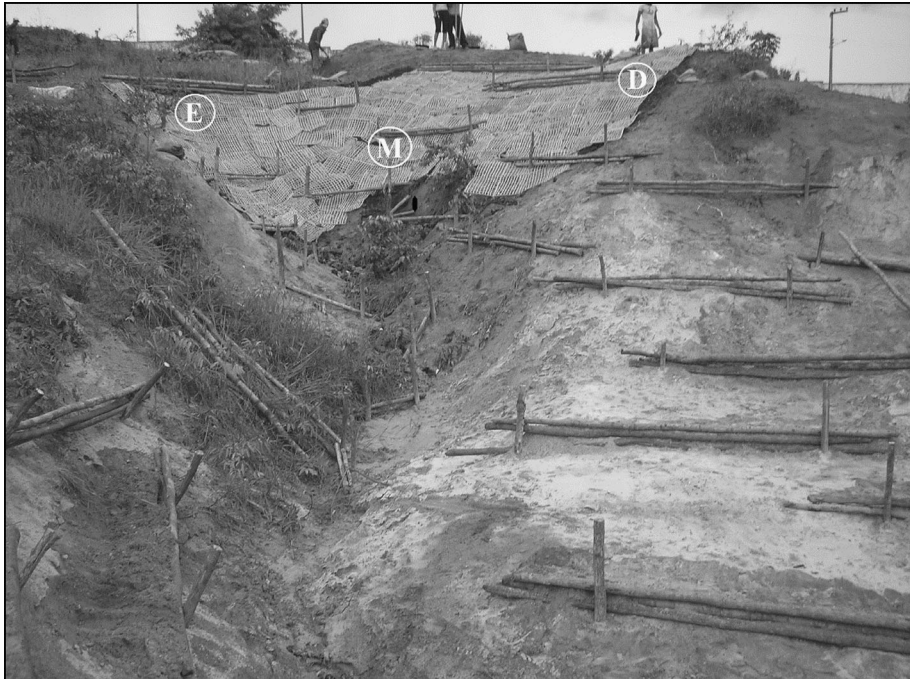
Fig. 2 Area 3 of the rehabilitated gully, with work in progress. E , M and D were reshaped exclusively by manual labour, São Luís, Brazil (LAGESOLOS 2008)
